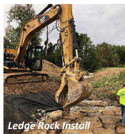
Streambank Stabilization
